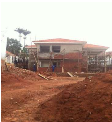
MoJCA Regional offices in Mbale under construction
