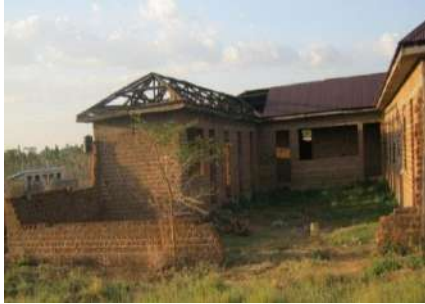
Pader Police Station - before
