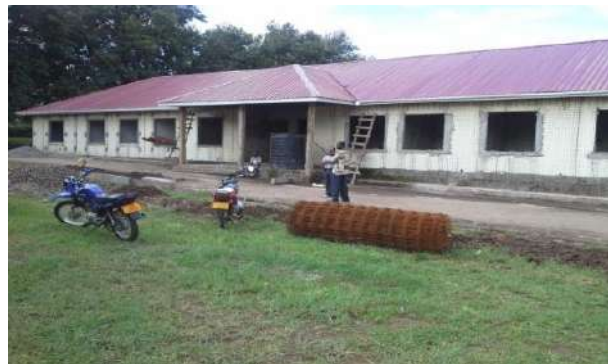
Moroto Station - After
