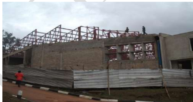
LDC auditorium under construction
