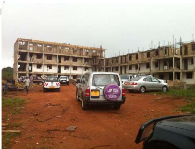
Kabalye PTS multi classroom block under construction
