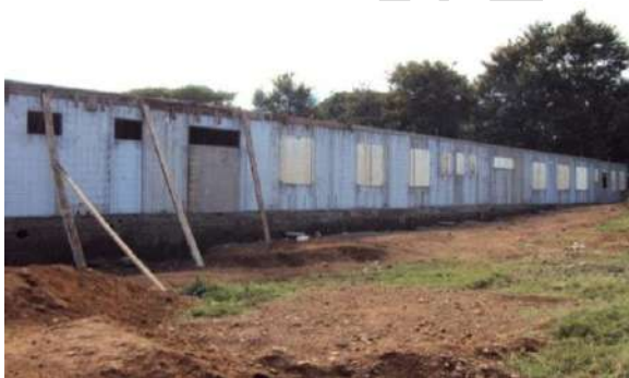
Moroto Station - Before
