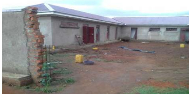
Pader Police Station - after
