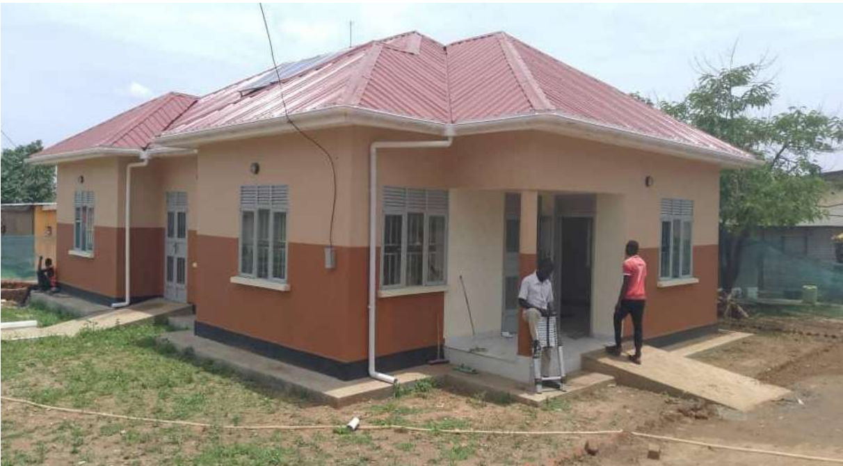
The newly constructed child reception center in Arua.
