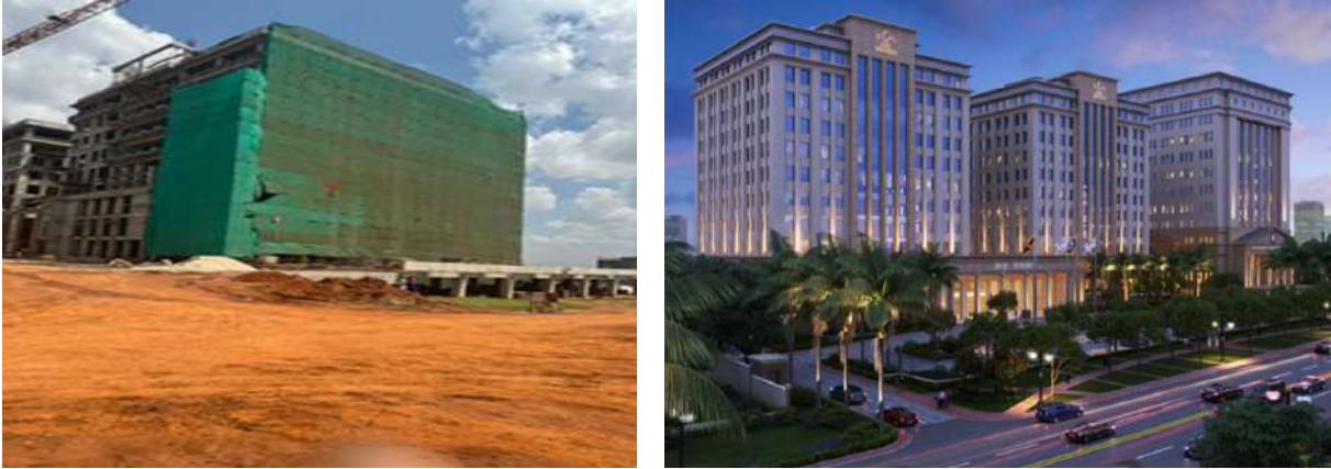
Ongoing construction and the artistic impression of the JLOS House
