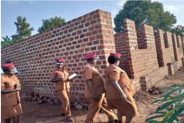
Staff houses constructed in Ngogwe Prison
