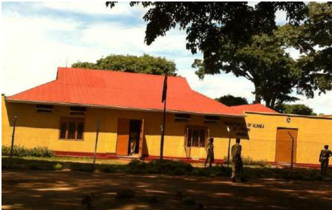
Amuria prison after renovation
